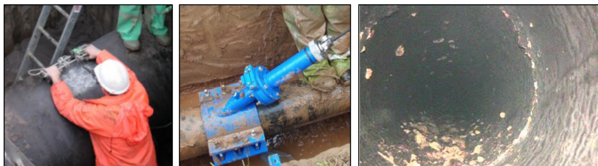
Figure 1: non-destructive testing of a trunk main
