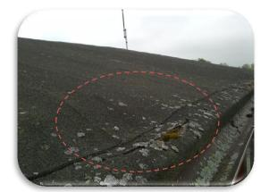
The roof lining on this building has deteriorated significantly during AMP5 and is causing incorrect rain water runoff. Interior leaks have been identified, damaging the interior walls. This roof has been acknowledged for investment in AMP6 in order to negate total roof failure. Preventative repairs have been made and its condition is being managed until refurbishment in AMP6.
