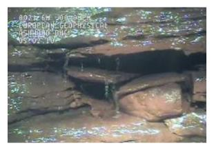
CCTV surveys in February 2010 have shown the existing boreholes to be in poor condition with fissures present at various depths.
