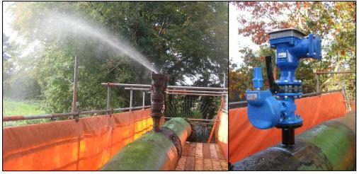
Figure 5: example air valve – pre and post intervention
