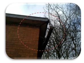
Example **R1** is a flat roof at a booster station, which during a building survey was found to require a significant refurbishment of the membrane and soffits. Minor remedial repairs have been made in order manage its condition throughout AMP5, to allow for refurbishment to be undertaken in AMP6.
