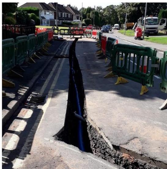
We also started work on a £450,000 programme in West Bromwich to replace 3km of cast iron mains, some of which are more than 65 years old, with more flexible and durable plastic pipes, which are less likely to crack and burst. We used innovative trenchless techniques for this scheme, which meant less digging and less inconvenience to local residents. And in September, we started work with our partners OnSite on a 20-week programme to upgrade more than 3km of water mains in Chase Terrace.
