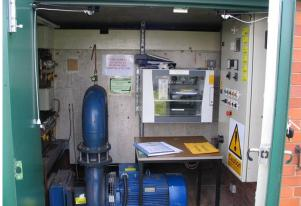
Images above show Hampton Loade's high lift pump hall at 12 MW of installed pumping capacity, and a small distribution booster of 30 kW capacity. Both of these sites would be treated equally in the booster stations per length of main variable, counting as one site each, which is clearly not reflective of the power costs nor the capital maintenance requirements.
